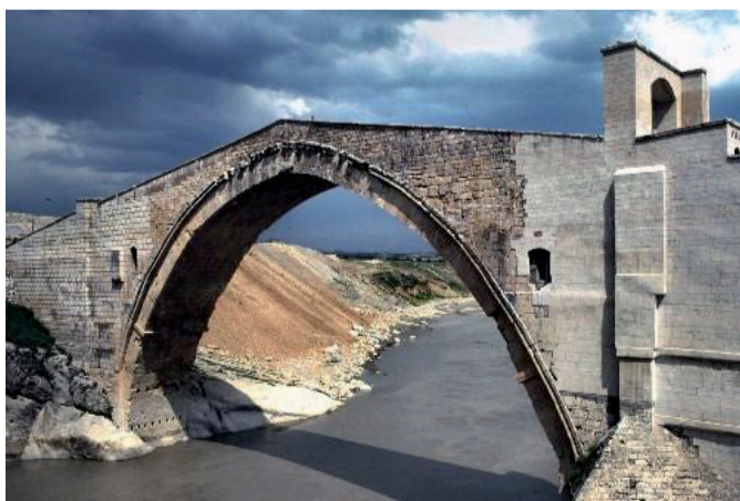
Fig 1.3.10. Malabadi Bridge in Diyarbakir
