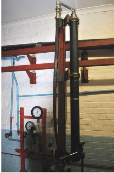
Figure 4-1: Photograph of the settling chamber in its 'open' position
