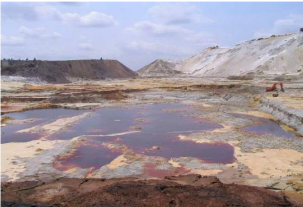
Figure 1.1: AMD formed owing to interaction between water and mine residue on the surface tailing reclamation operation in the Western Basin. This site drains into pit operations that are directly connected to mine void
