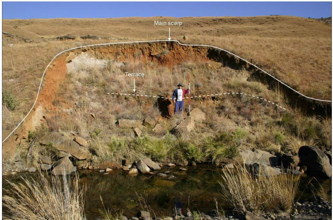
Figure 6.26 Oblique photograph of the translational slide at site I on the Bushman's River.
