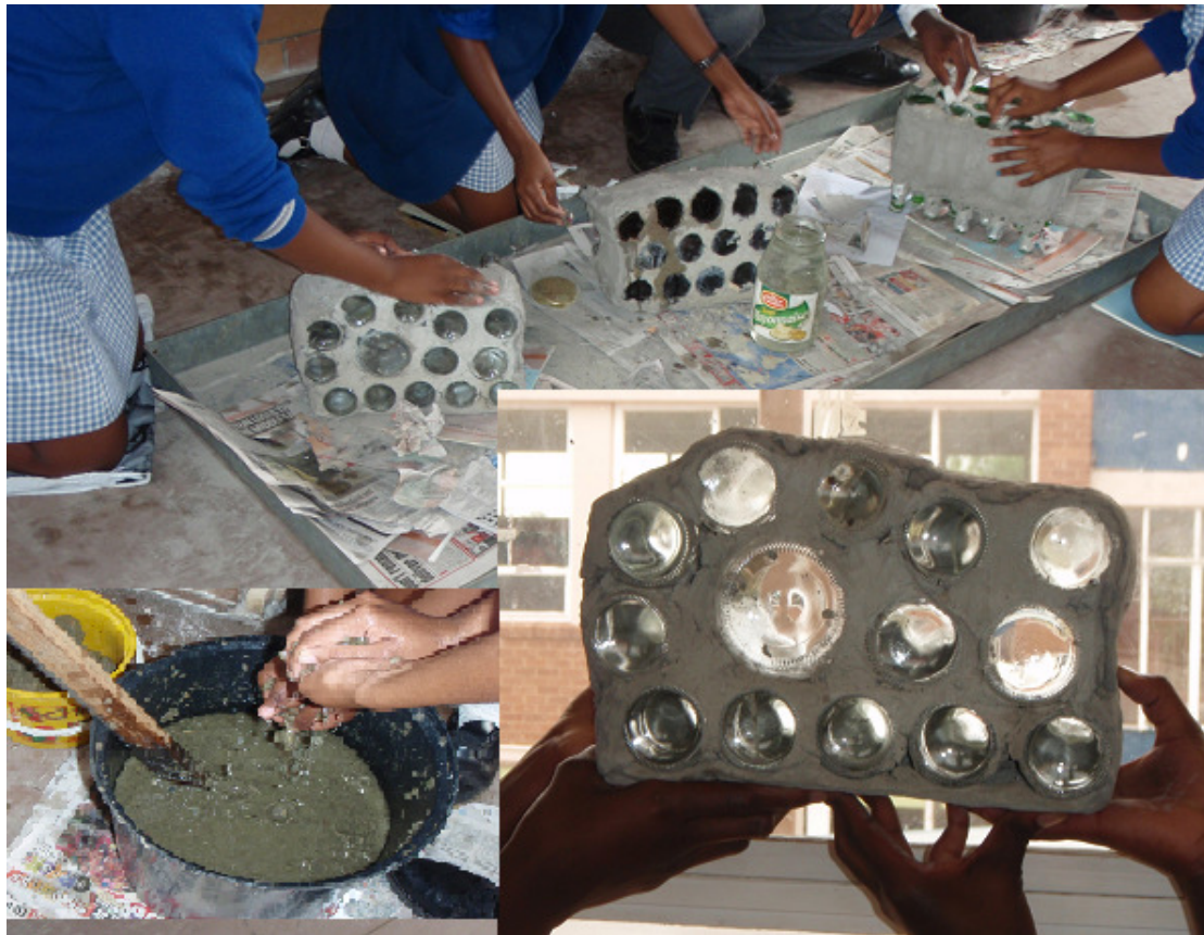
Figure 4: Eco brick production
