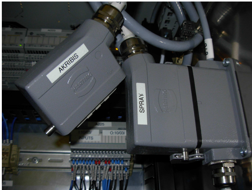
Figure 4.2: Test Stand Injector Current Plugs
