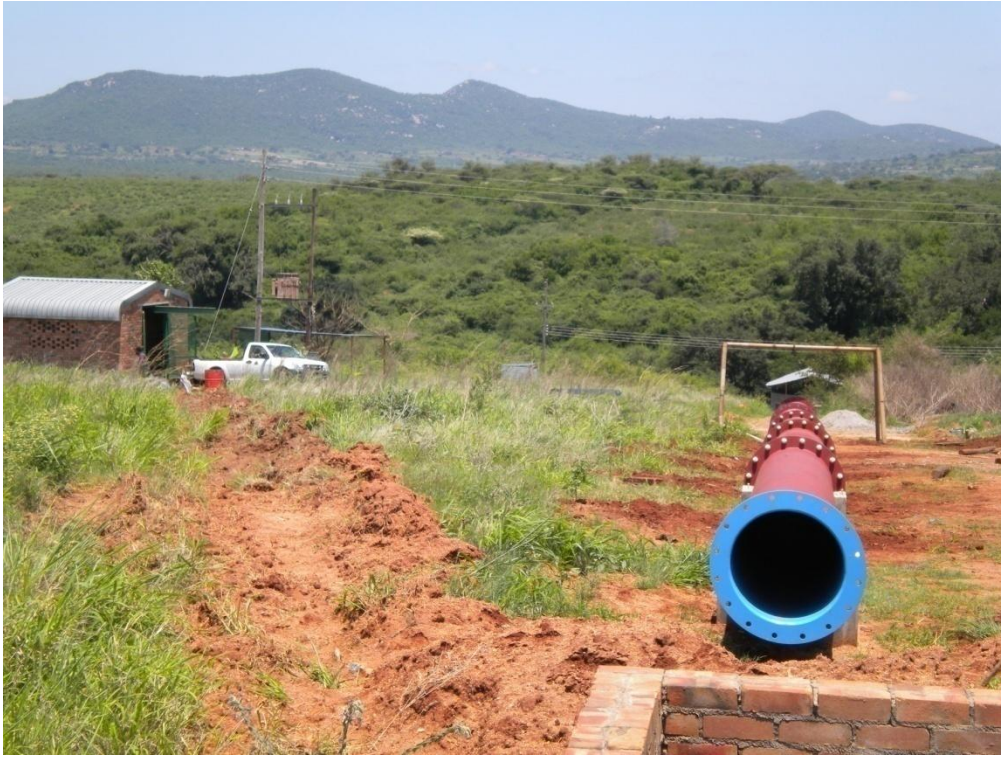
Figure 7 On-going irrigation rehabilitation works at Vuka Shidwashini
