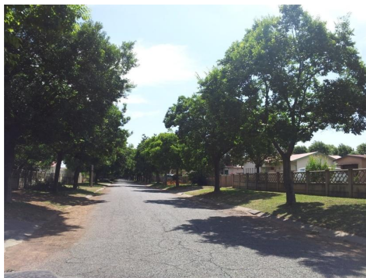
Figure 14: A view of a typical street where the field tests were carried out in Vanderbijlpark (Area B)
