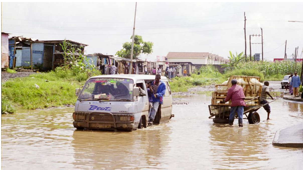
Figure 4.2: A section of a desperately in need of maintenance road in Nairobi's Eastlands in the 1990s (photo Courtesy of Antony Kaminju).
