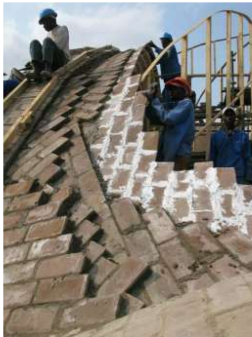
Figure 2: The Mapungubwe Interpretation Center during construction (compliments from Dezeen Limited)
