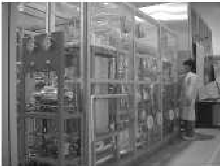
A pilot plant using ozone to destruct organic waste in Japan. (Fukasawa, et al., 2001)
