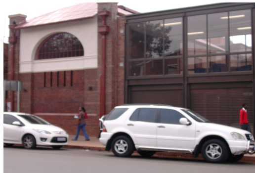
Old Tram Shed converted into a new library
