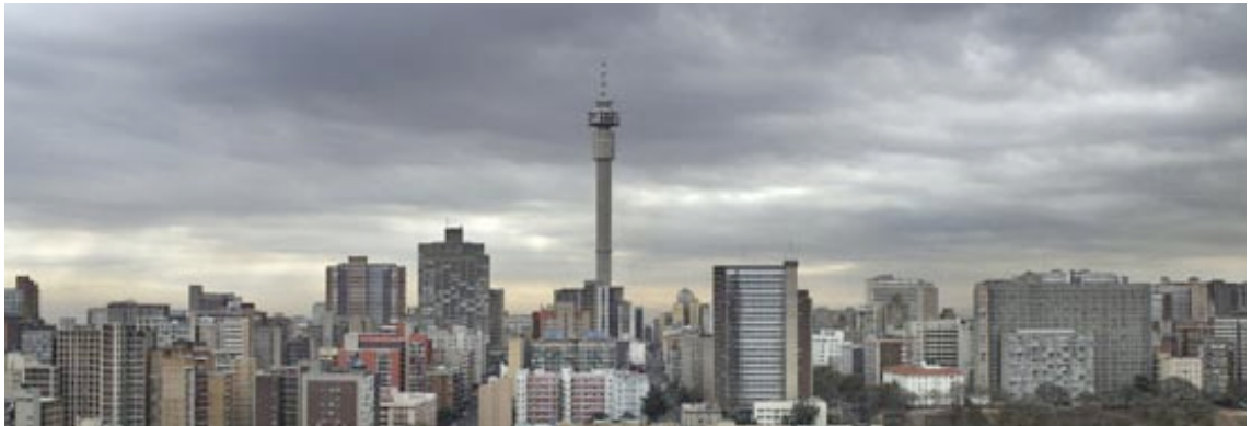
Guy Tillim, (Detail) View of Hillbrow looking north from the roof of the Mariston Hotel , 2004
