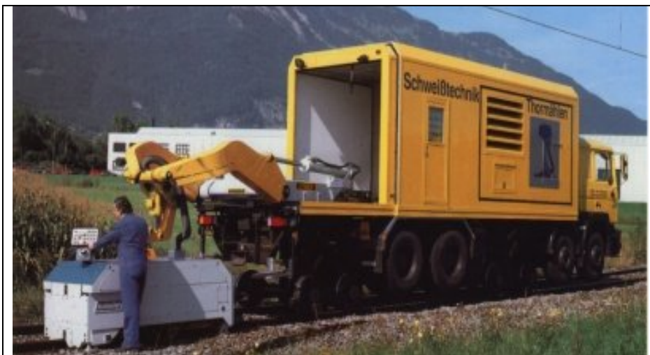
Figure 2.8: Combined vehicle rail/road for flash butt welding
