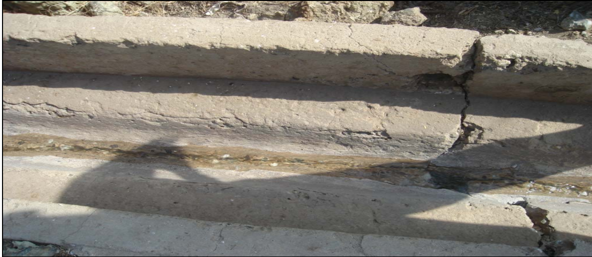
Figure 4.8: Clean water flowing in a surface water run-off drain
