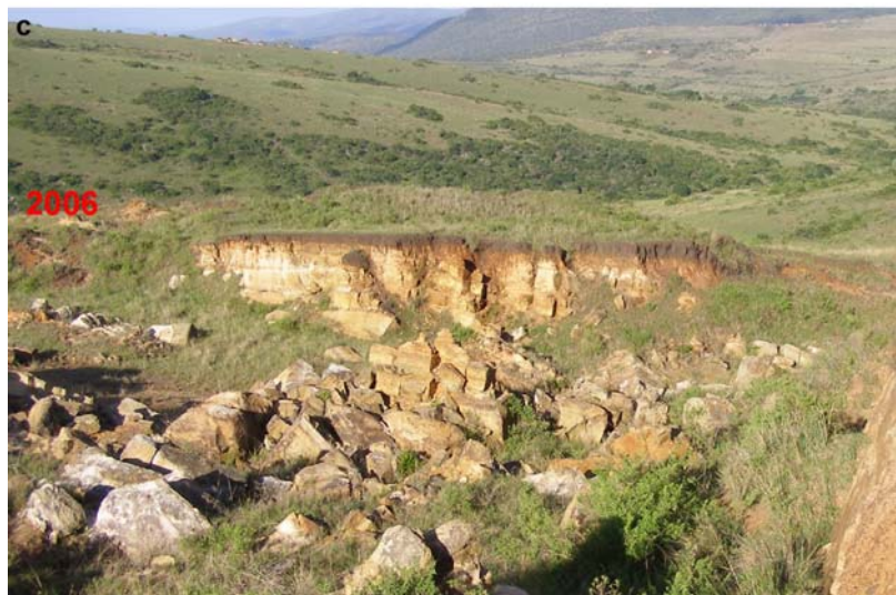
Figure 10a-c. (a) A translational slide occurred in the sandstones of the Vryheid Formation on an eastward facing slope in the Molletshe Tribal Authority area in 1991. (b) View of the translational slide in 1991 showing sharp morphological landslide features. (c) View of the slide in 2006 showing similarities in the morphological landslide features since the landslide event.
