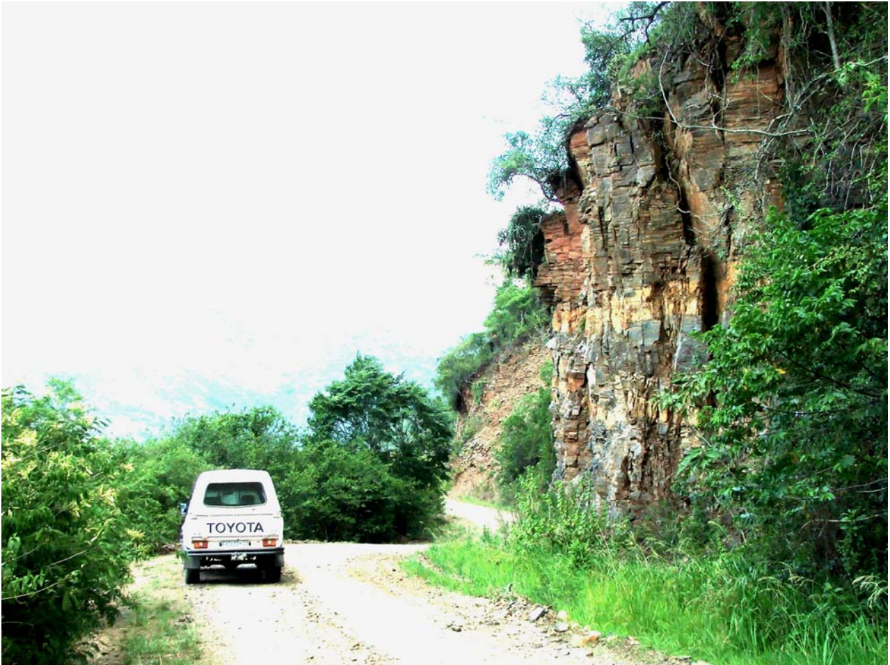
Figure 36. Toppling in vertically jointed shales in the vicinity of Helehele.
