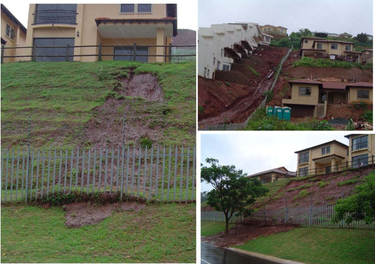
Figure 38. Shallow flows associated with the “Berea Red Sand” in the La Lucia area, north of Durban.
