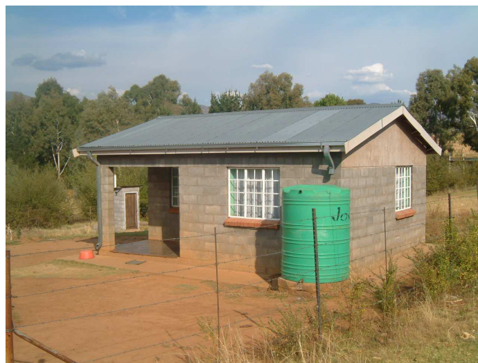
Picture 7-7: LHDA constructed house in Ha Nazareth (2007)
