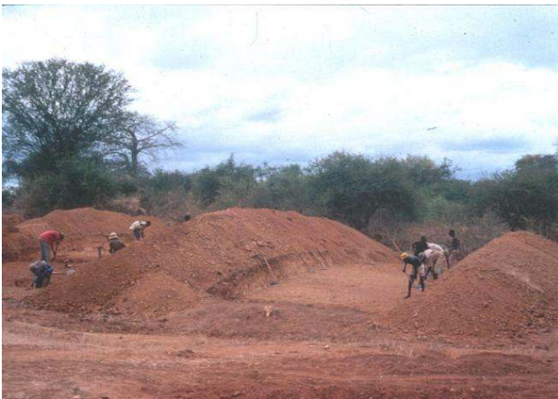
Fig A1-2: Quarry, Rural Access Roads Programme, Kenya. (Photo: RT McCutcheon)
