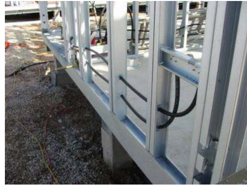
Fig 5-16: Completed framework (Group5 2007) Fig 5-17: Flexible conduit (Group5 2007)
