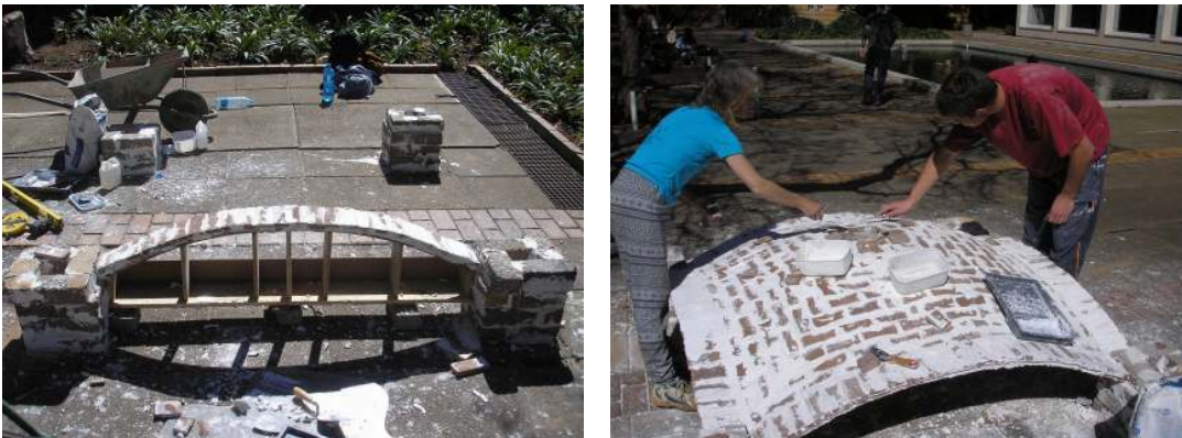
Fig 6-15: Timbrel vault, scale 1:4
