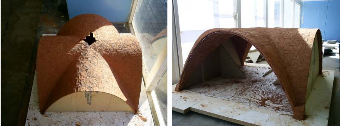
Fig 6-21: 1:10 Catenary groin vault under construction
