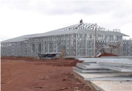
Fig 5-16: Completed framework (Group5 2007) Fig 5-17: Flexible conduit (Group5 2007)
