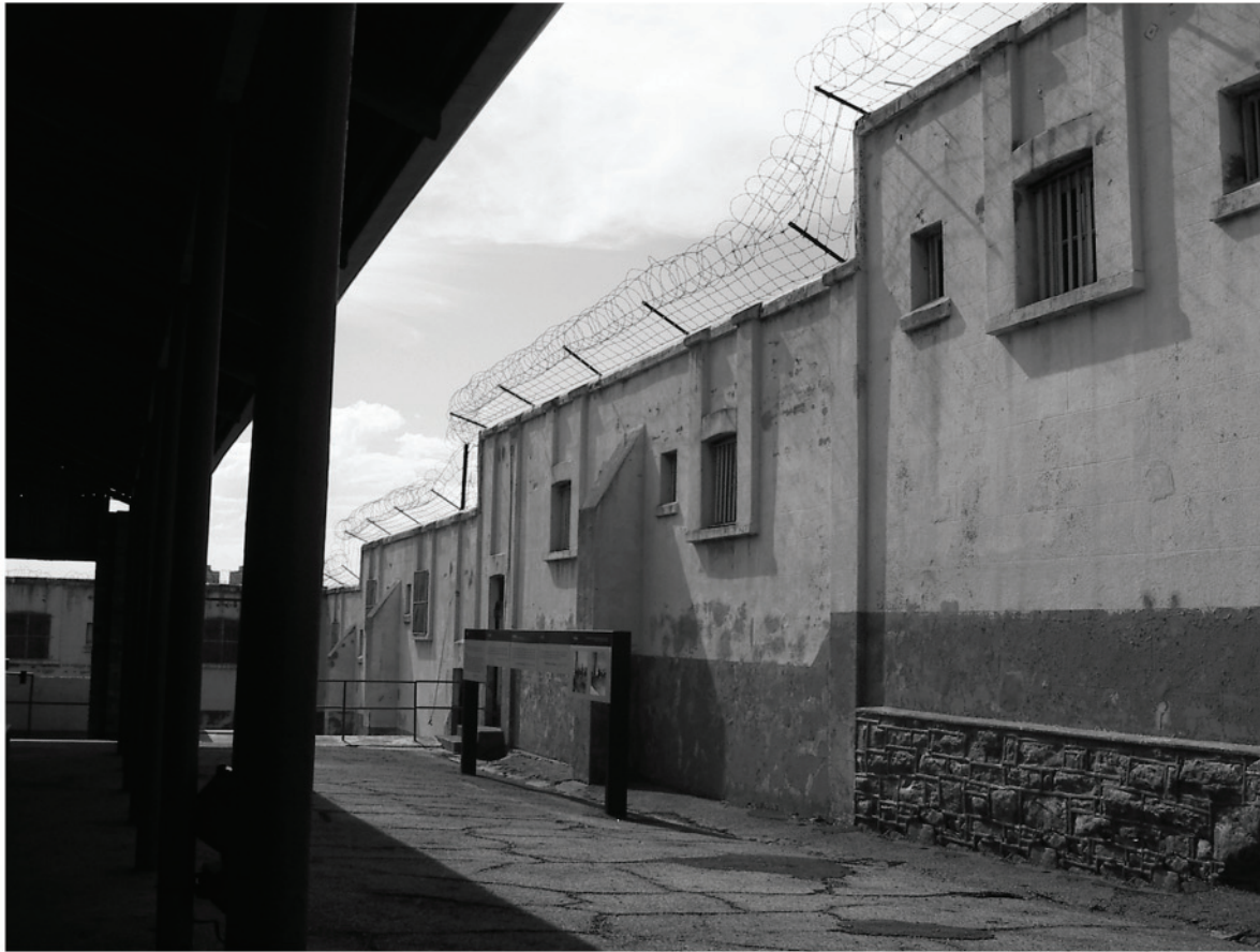
→ above: view of prison wall at the 'Old Fort', Constitution Hill.
