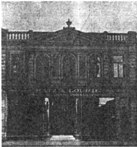
The Commissioner Street shop (1911)
