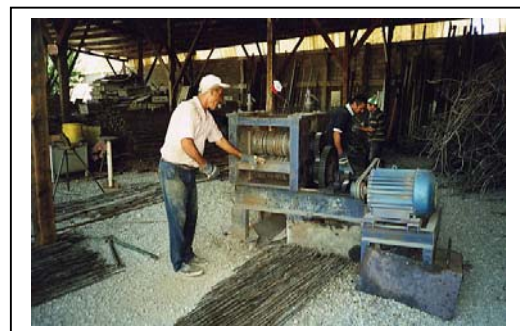
Figure 26: Processing of recovered steel reinforcement, Turkey.
