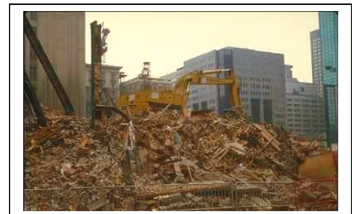
Figure 7: Rubble from a demolished building mainly mixed debris
