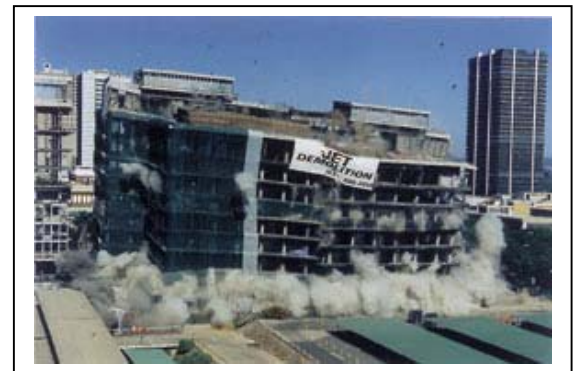
Figure 3: Demolition with explosives
