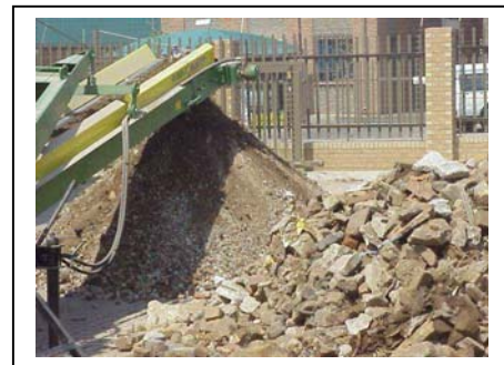
Figure 17: Rubble recycled to fill material
