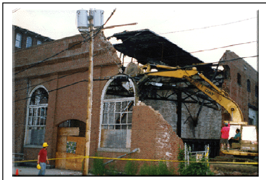
Figure 2: Demolition with plant
