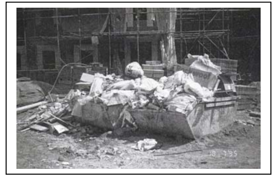
Figure 5: The use of single receptacles, which fill up quickly and take long to be emptied
