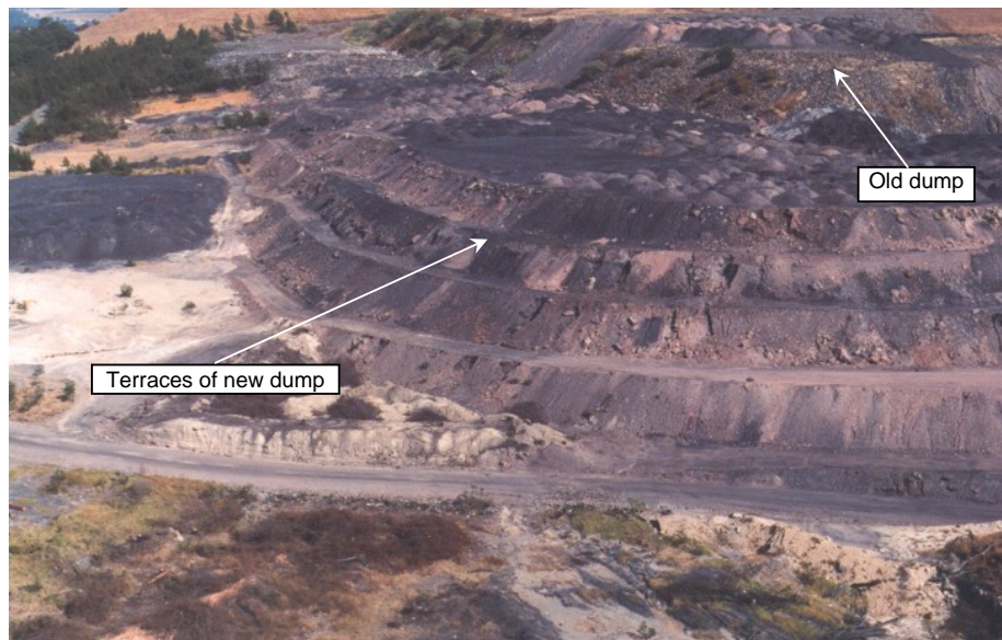
Figure 4.3 Extension of Dump No.2 by keying in material from Dump No.1 in compacted terraces.
