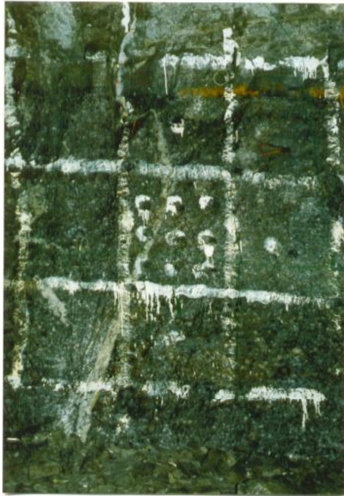
PHOTOGRAPH 9.3 SHOWING 9 – HOLE BURN CUT
