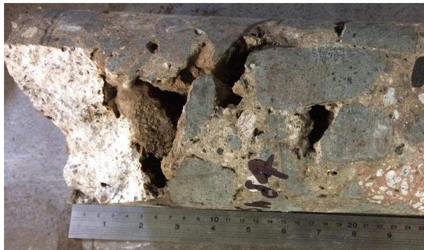
Figure 6-40 – Large air voids from poor compaction in Sample 84
