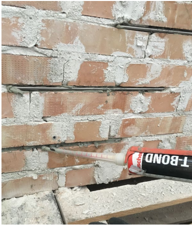
Figure 17: A repaired wall panel using titanium rods for crack stitching.
