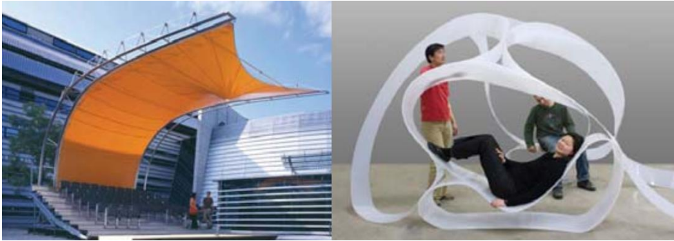
Figure 28 - Strut and cable braced cantilever, Munich, UK, 2002 (left); LOOP, New York, 2006 (right).
