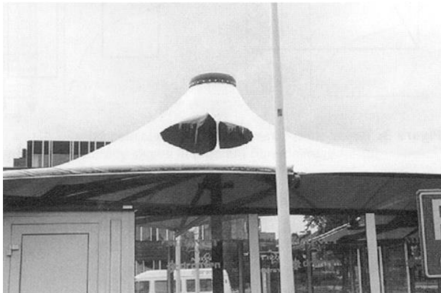
Figure 10 - PVC coated Polyester structure in the Netherlands after local fire a hole occurs in the membrane, but the fabric itself is not destroyed. (Houtman and Orpana 2000)
