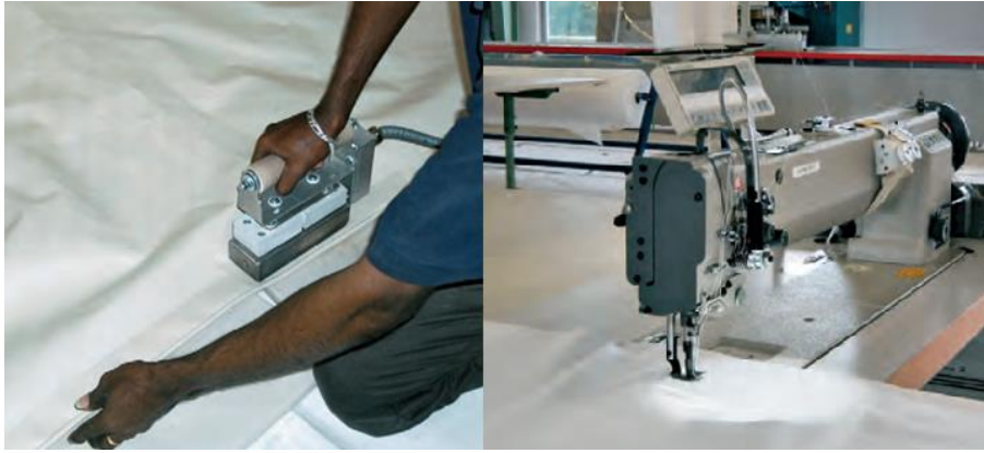
Figure 23 – Jointing processes. Manual welding device (left), industrial sewing machine (right).
