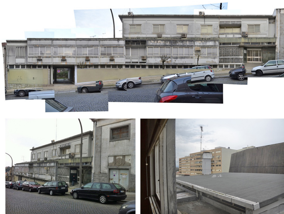
Figure 7. Current state of the Abade Loureira building
