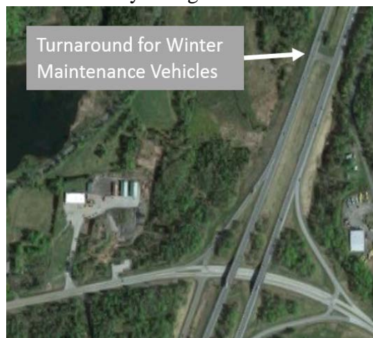
Figure D.4. Winter maintenance vehicle turnaround near Interstate 89 Exit 5, VT
