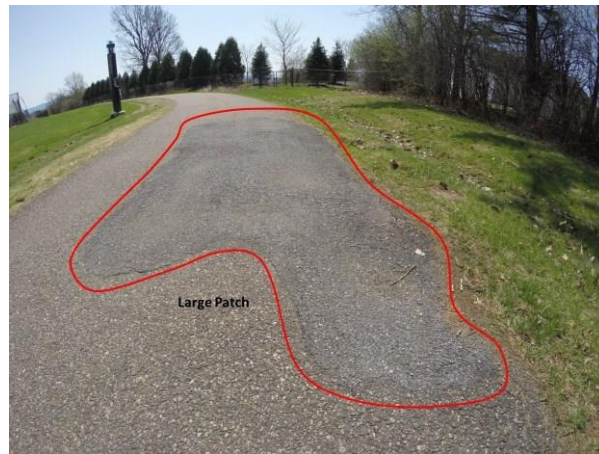
Figure 53 Test Spot with Large Asphalt Patch
