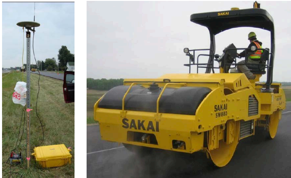
Figure 4. GPS system for the IC earthwork constructions (Source: Naras et al., 2015)
