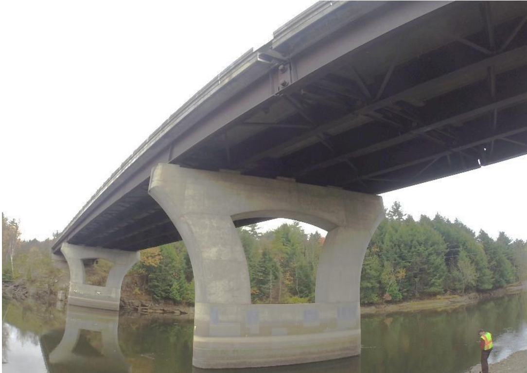
Figure 5.18 US 2 Lamoille River Crossing Bridge with hanger pin joints
