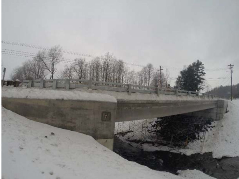
Figure 36: Full View of Gold Brook Bridge in Stowe (12/18/14)
