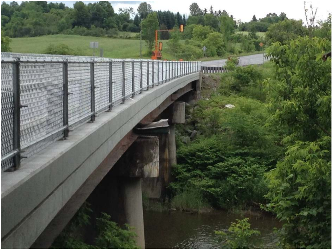
Figure 4.6 US 7 New Haven Br. #129 – REPAIRED Fascia/Curb Reconstruction, $350,000
