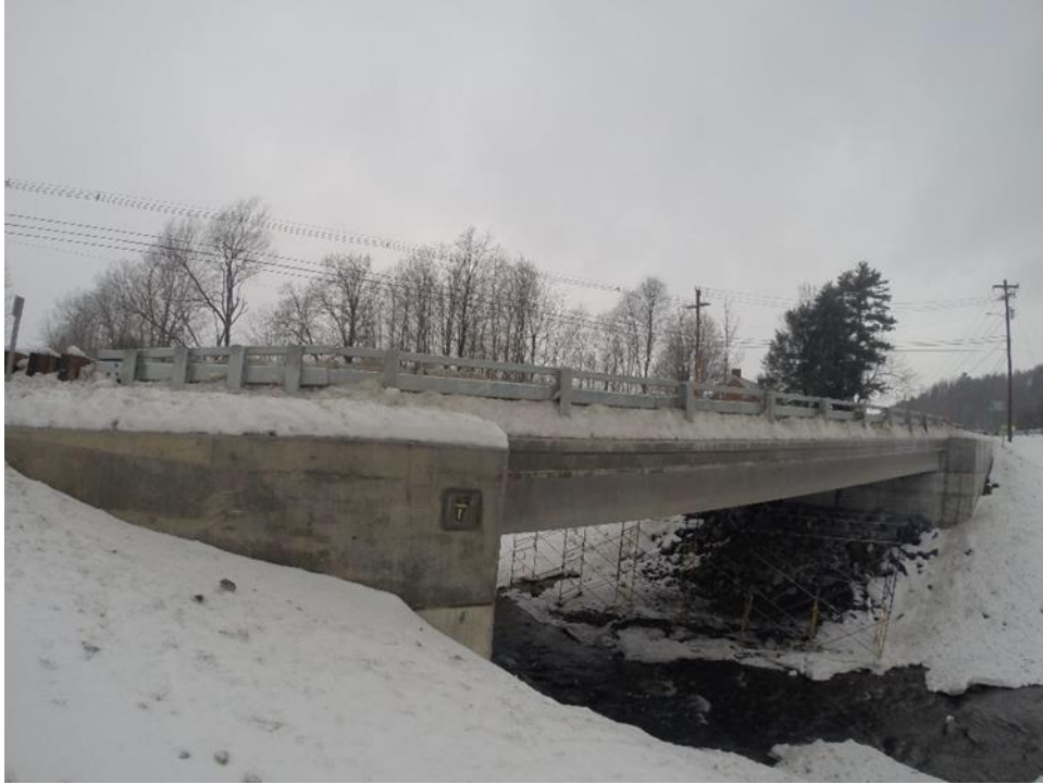
Figure 5.41 Stowe Rte 100 Gold Brook Crossing Bridge
