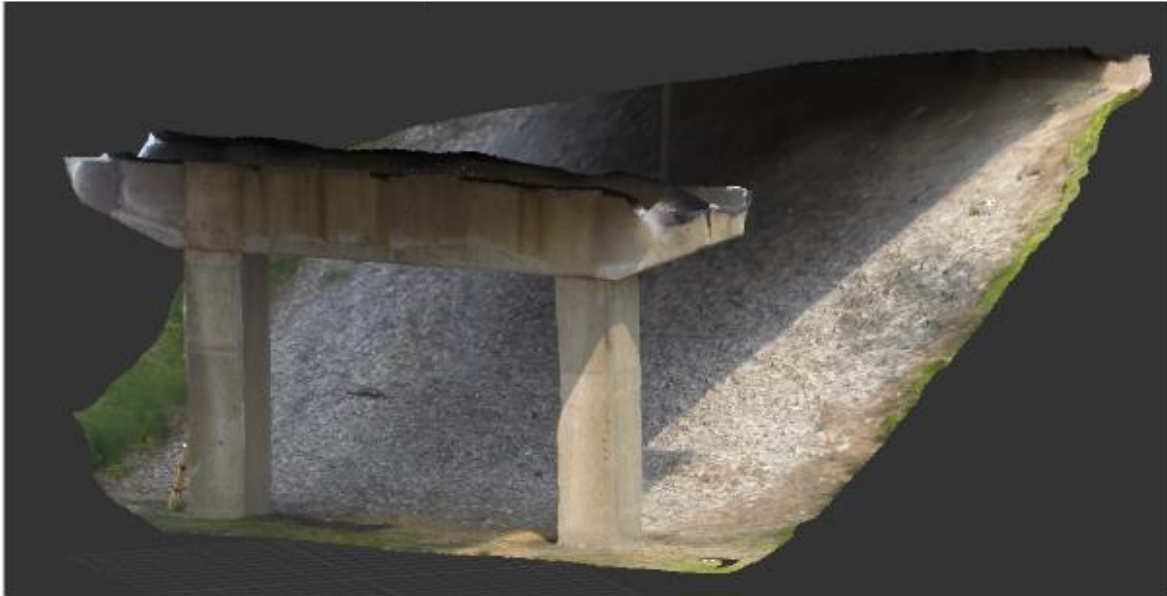
3D Cloud point data of Pier 1 in Auto Desk RECAP PRO
