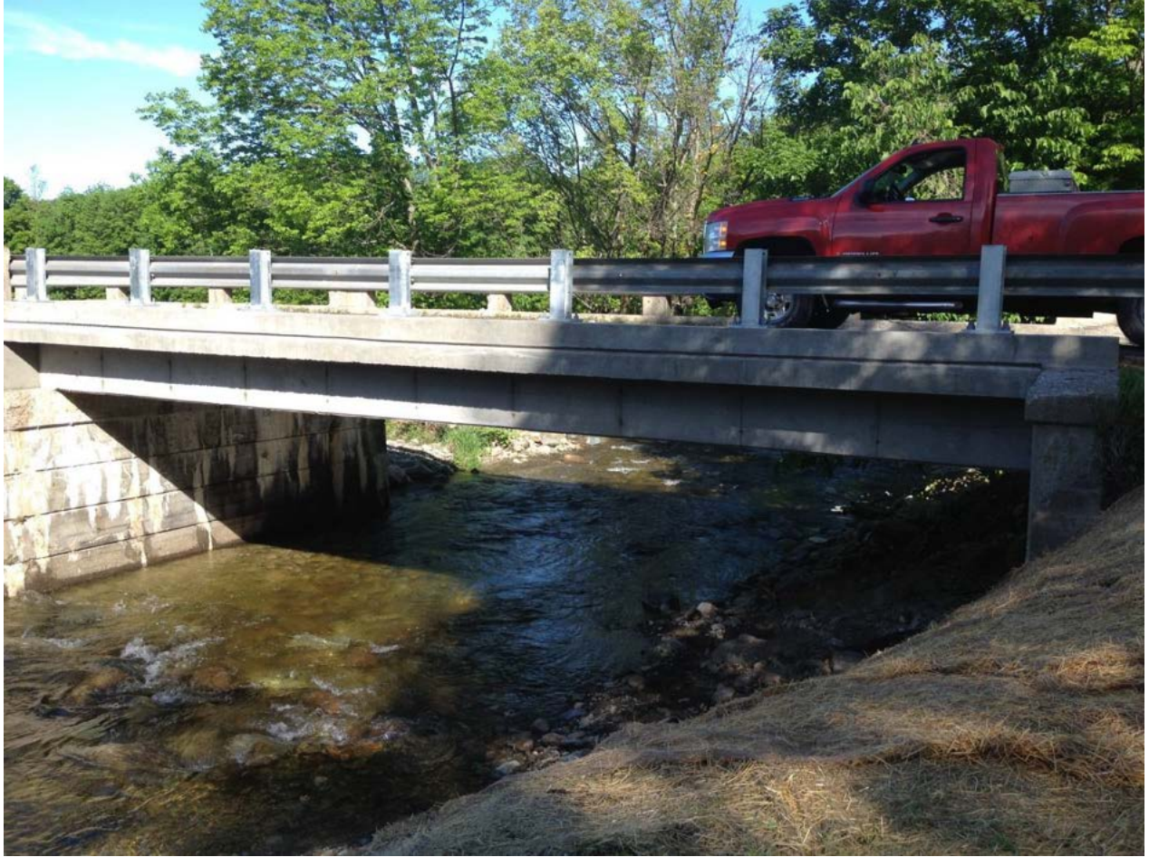
Figure 4.24 Vt. Rte. 105A Richford Br. #2 –REPAIRED T Beam/Deck Reconstruction $150,000
