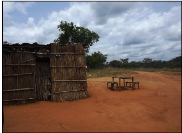
Figure 29 – House in the DSA. Straw walls and roof
