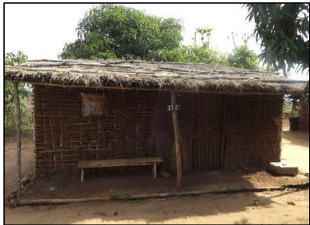
Figure 31 – House in the DSA. Wattle and daub walls, straw roof, and earth floor.
