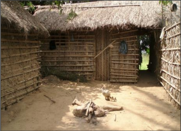
Figure 41 – Houses without a kitchen
