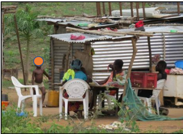
Figure 30 - House in the DSA. Iron sheet walls and roof.
