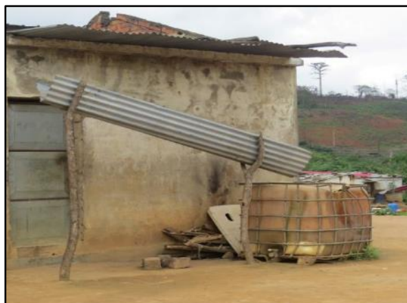
Figure 35 –Water sources – Unprotected tank
