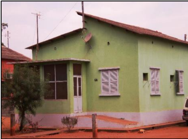
Figure 26 - House in the DSA. Block walls and fibrocement roof
