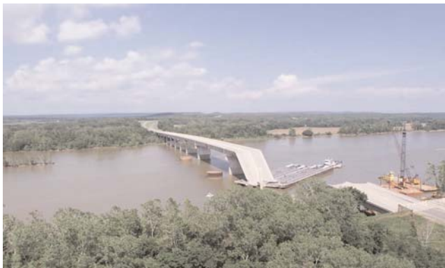
FIGURE 2 Overview of damaged I-40 Webbers Falls Bridge.
