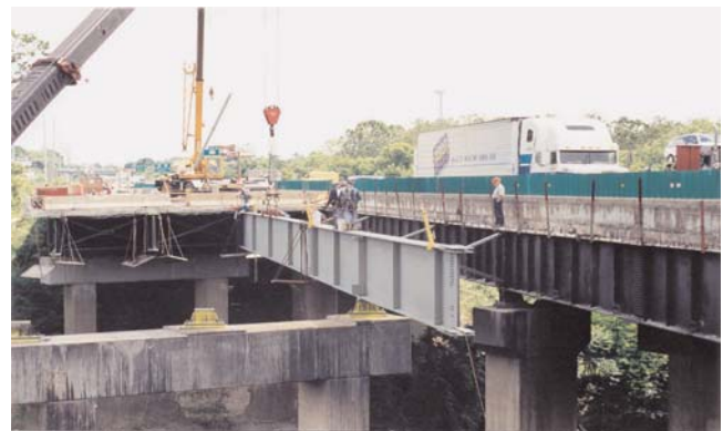
FIGURE 3 Reconstruction of I-95 southbound bridge and temporary detour lanes.
