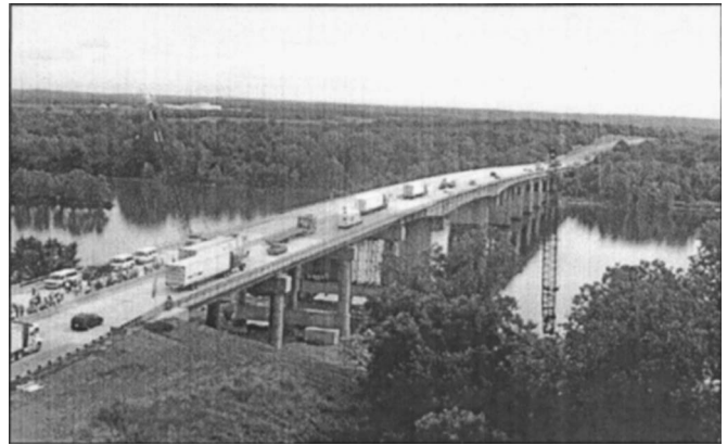
Fig. 5. I-40 bridge reopened to traveling public
