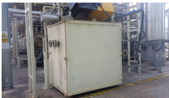
Figure 5. Photo of the final part of the process line for the removal of contaminants from reactor R101. The K201 container with the PK201 feeder can be seen in the foreground.
