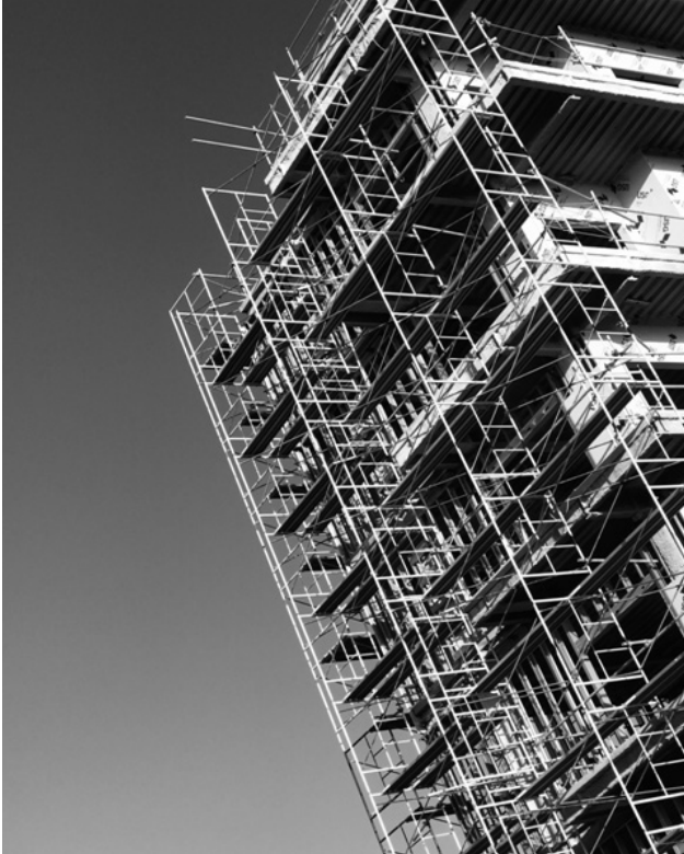
Figure 10. 'Progress': Construction Site in Aruba © Hannah Mayr.
