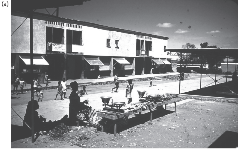
Figure 3.11a: Two-story housing with shops for commercial activities on the ground floor. Notice the informal infrastructure for selling food in the front, situation late 1950s. Source: contemporary original color slide, AA, Ministry of Foreign Affairs, Brussels; Fund OCA, Courtesy AA.
