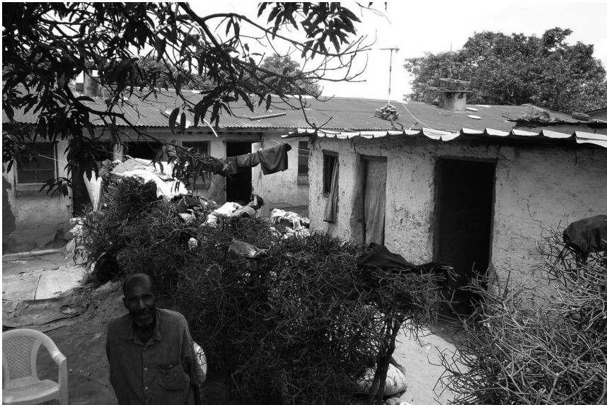
Figure 3.14: Transformation of an OCA house with an additional facility added to the back side. Source: photograph by Céline Fenaux, 2010.
