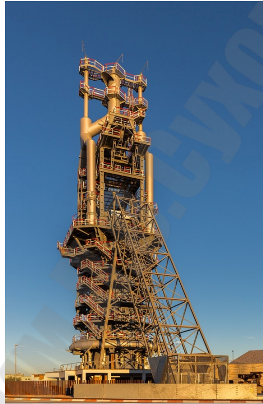
Blast furnace in Port of Sagunto, Spain
