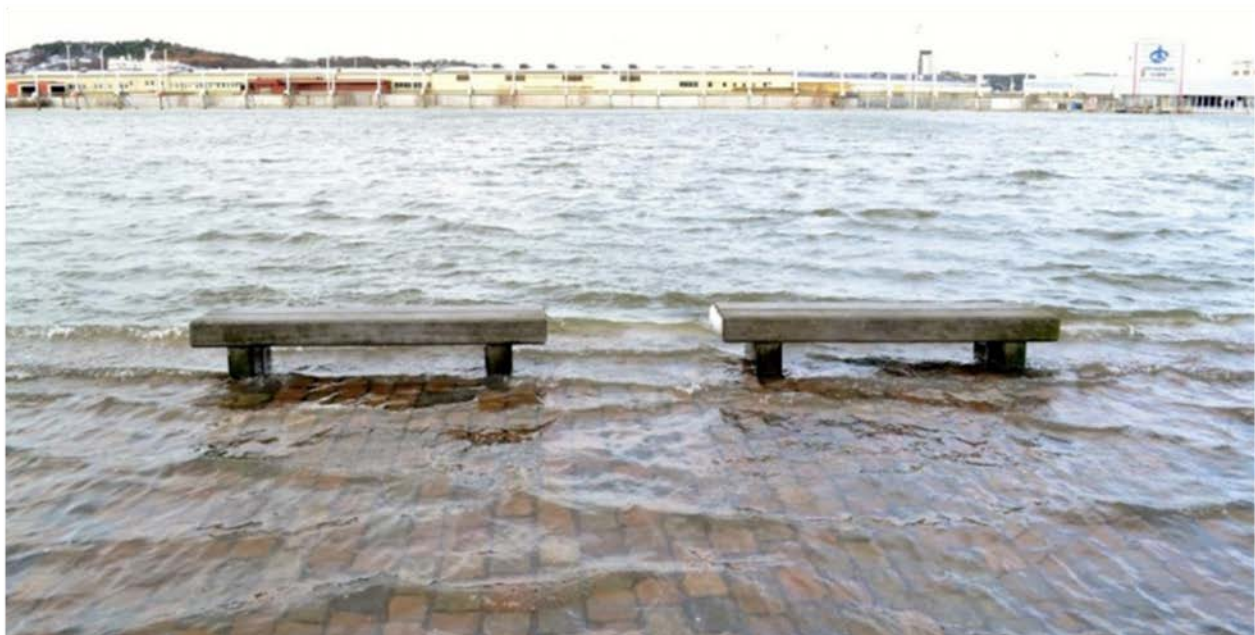
Figure 1: Increased sea level in river Göta älv, behind the Opera House, due to the storm Sven that struck Gothenburg in December 2013. Photo: Susanna Gelin
