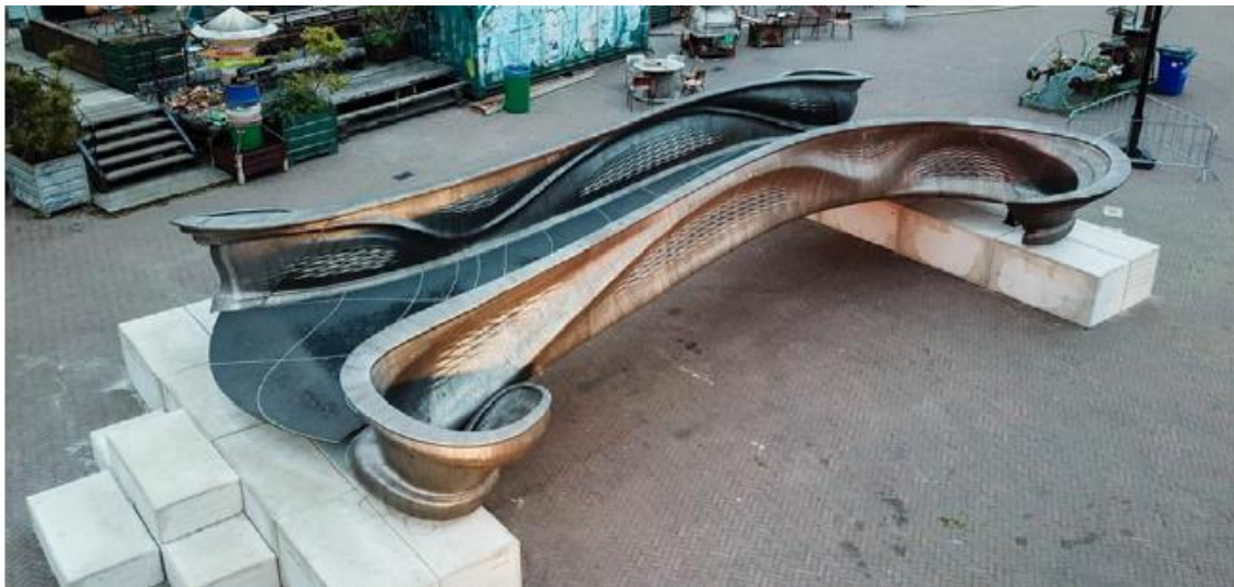
Figure 2-298 MX3D pedestrian bridge[?].
