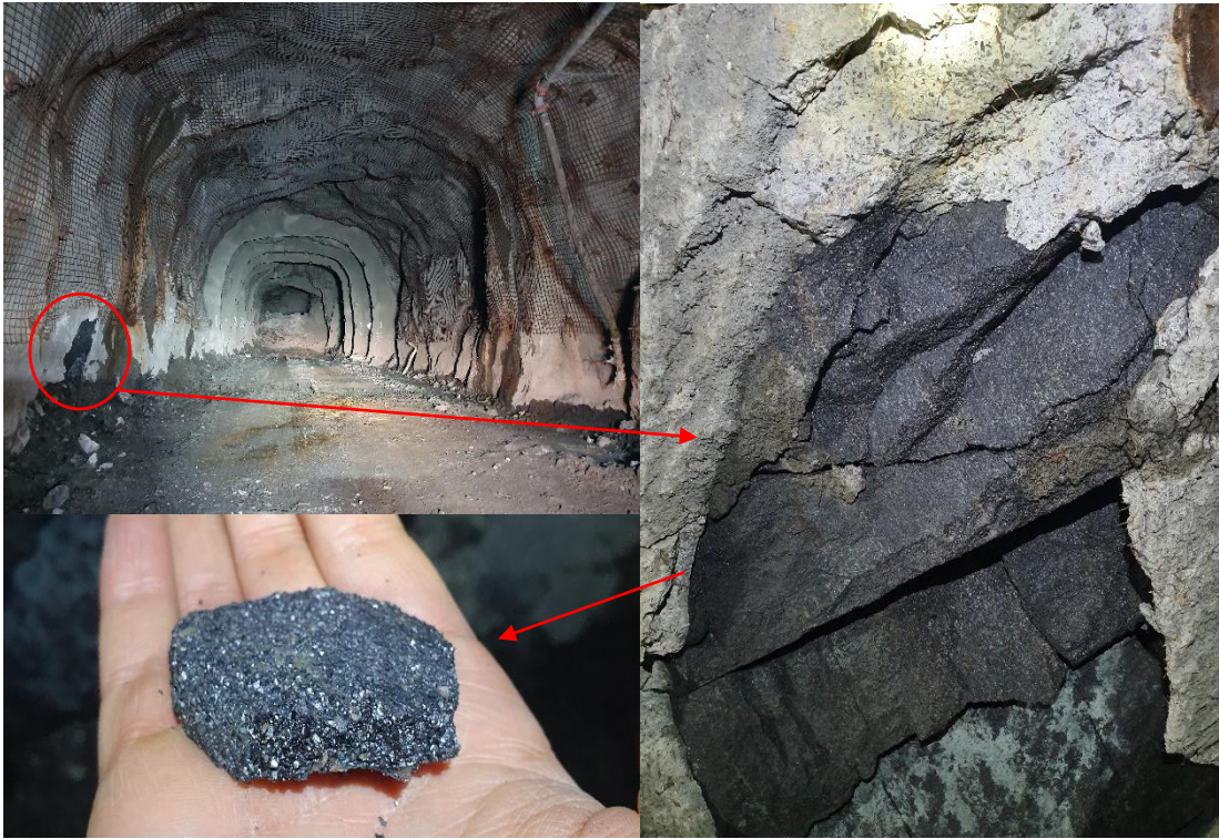
Figure 28: Current state in HO1051o2730
