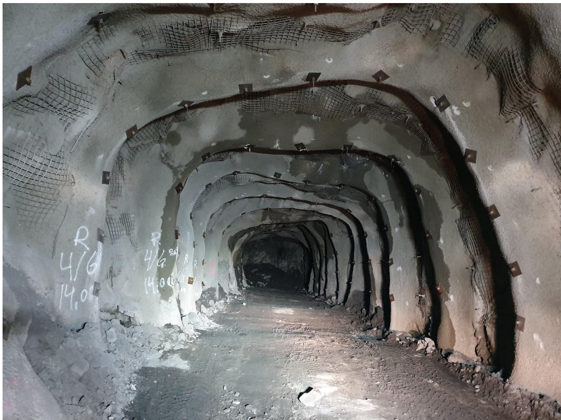
Figure 14: Crosscut PR996, 4110 with installed fibrecrete arches
