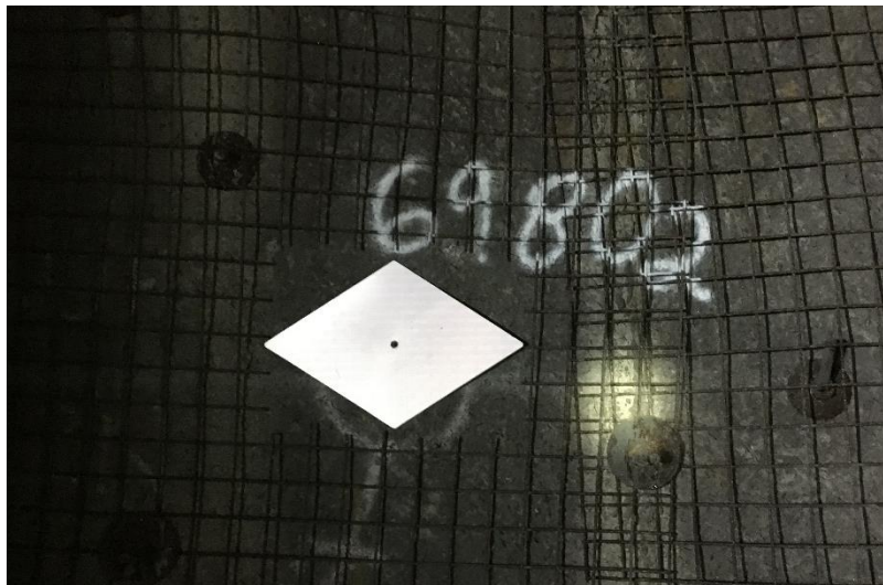
Figure 37: LiDAR target installed in a drift
