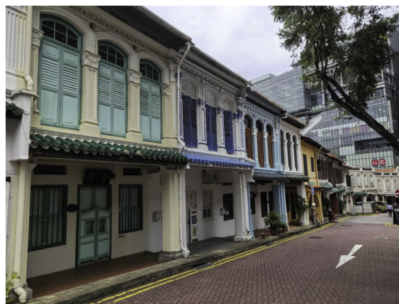
Fig. 1. Emerald Hill, a neighborhood with Straits Chinese style of 'Chinese Baroque' terrace houses, conserved in 1989.
