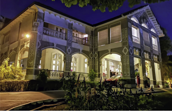
Fig. 2. Eden Hall Bungalow at Nassim Road, a colonial bungalow that serves as the British High Commissioner's official residence in Singapore, was conserved in 1991.
