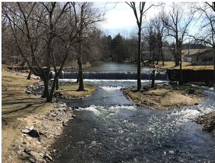
Figure 2. Roller Mill dam on Chiques Creek near Manheim, Pennsylvania (view looking upstream). The height of the dam is around 2.4 m and was originally constructed in the 1700s and rebuilt several times thereafter. Note the sharp difference in stream water levels above and below the dam.
