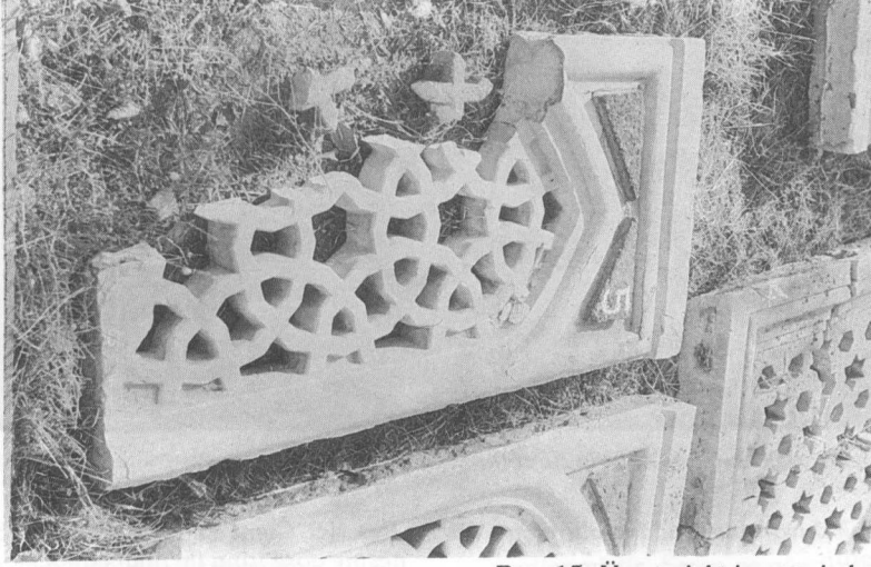
Res. 15: Üzerindeki boya tabakası çözücü solventlerle yumuşatılıp kaldırılan künde-kari pencere kepenklerinden biri. (One of the window shutters of the künde-kari window, which has been softened and removed with solvent on the paint layer.)
