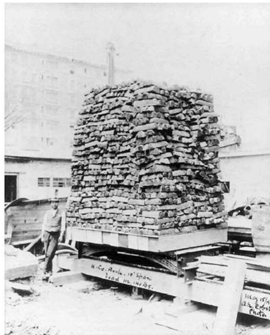
Fig.1.4. Static load test carried out by Rafael Guastavino (Guastavino/Collins archive. Columbia University).
