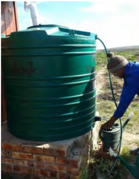
Figure 4: Resident collecting water from a community rainwater tank
