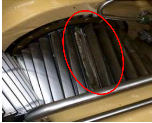
Figure 7. Wear on the gearbox.
