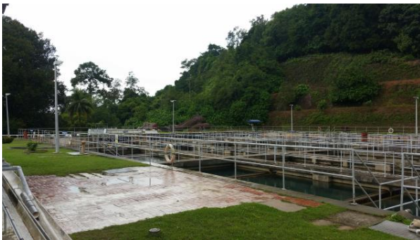
Figure 1. Water sedimentation plant.
