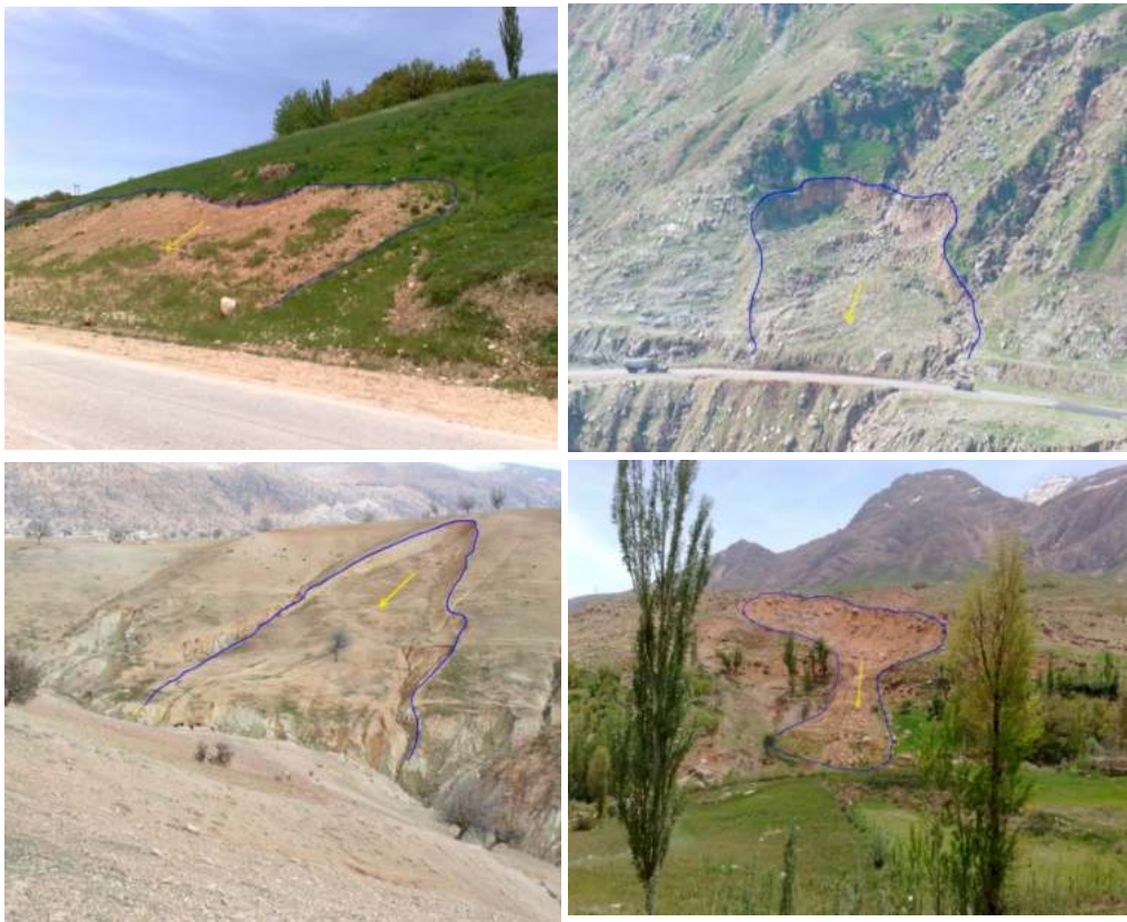
Figure 2. Some recent landslides in the Sarkhoon watershed.
