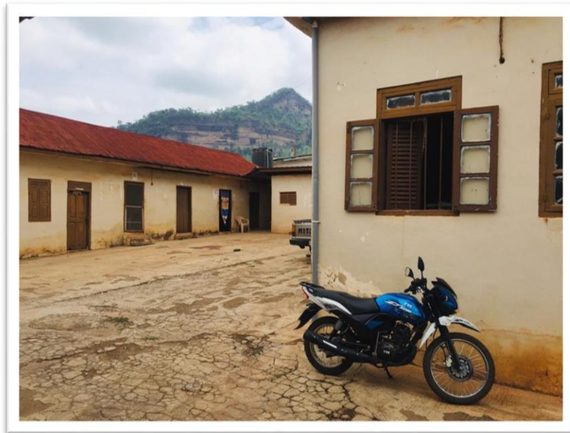
A District Health Administration office building in the Eastern Region of Ghana
